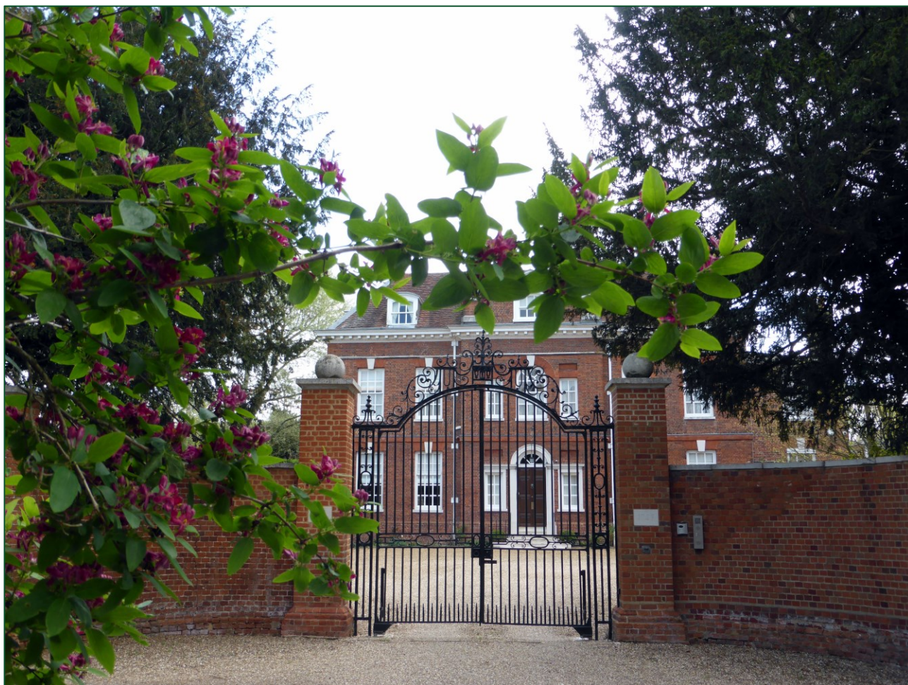
Figure 15 Permeable gates at Hadham Hall
